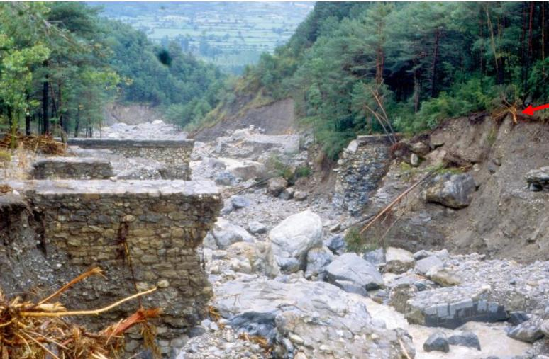
Most of the 40 check dams destroyed, releasing about 68,000 m<sup>3</sup> of stored sediments which spread over the fan. Channel with capacity of  $120 \text{ m}^3\text{s}^{-1}$  was overflowed and buried
