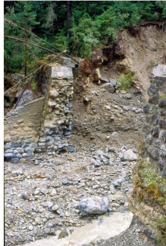
Causes of failure: dam undermining, scour of lateral support, hydrostatic pressure, impact of boulders
