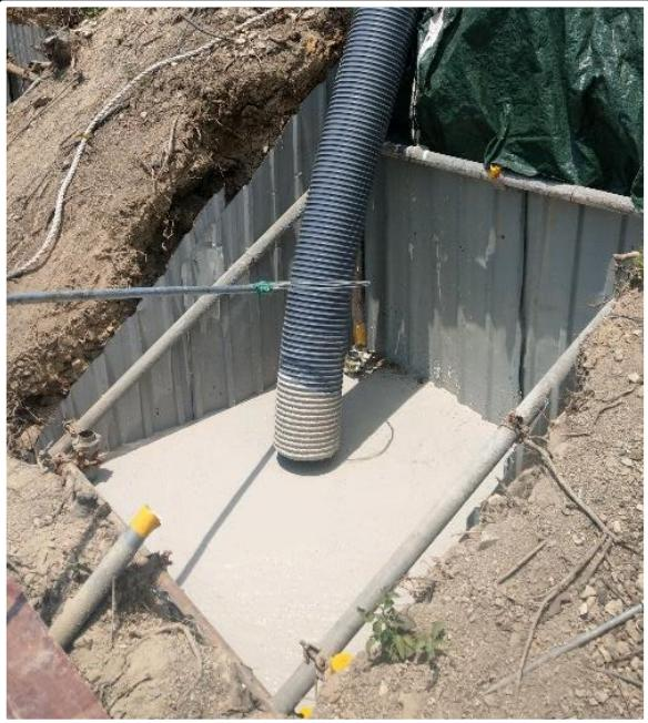
Self-compacting backfill material
